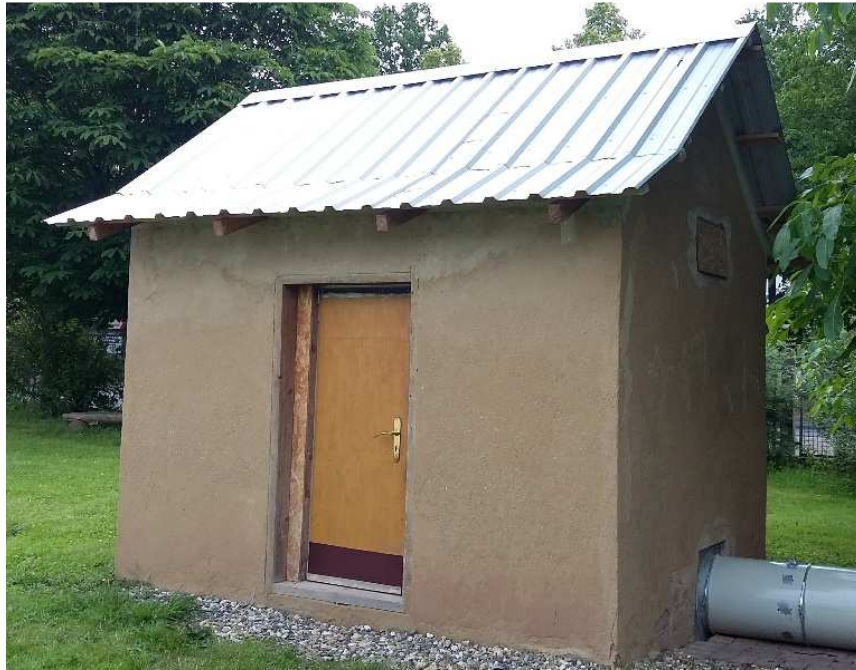
Figure 1-A Constructed mud storehouse.
