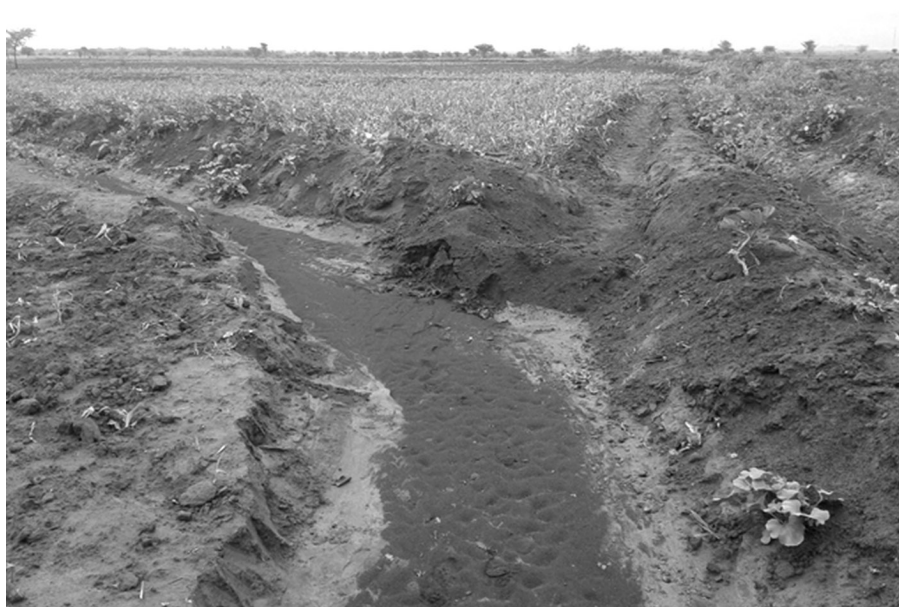
Fig. 4: Micro diversion bund at field level
